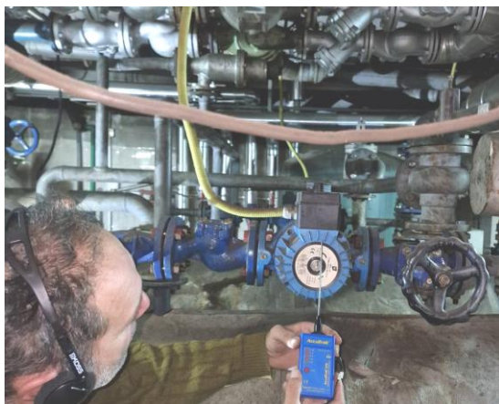
Figure 6 – Checking the wear of rotating pump parts in the gas boiler room
