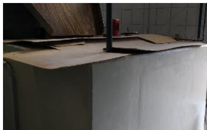
Figure 6 Sludge tank (source: author archives)
