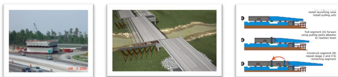
Figure 1: Prefabricated Bridge Units, Lateral Slide & Incremental Launching [13]
