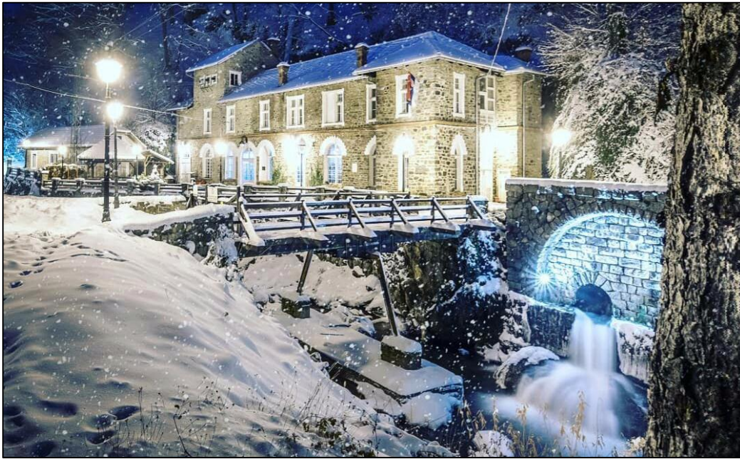
Image 1 – Hydroelectric Power Plant "Vučje" from 1903, on the Vučjanka River, near Leskovac, in Serbia
